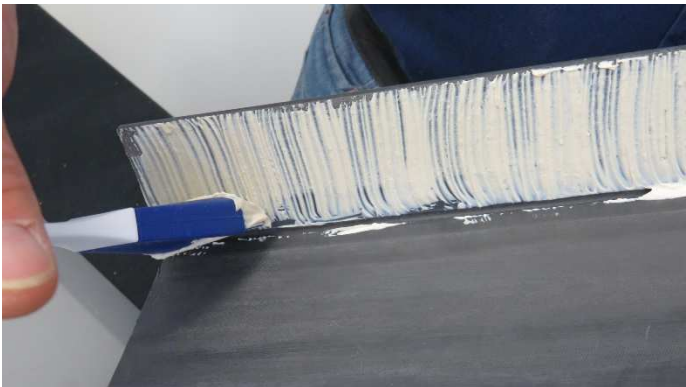
Using the slightly modified basting brush, apply the 946 adhesive to the back of the tread nose and to the face of the step riser. Applying the adhesive in opposite directions, will assist with the adhesive bond. 100% coverage on both the tread nose and step riser must be achieved.
